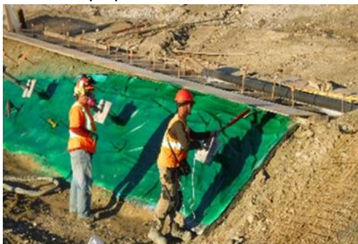
Figure 3. Spray applied PU liner on earthen berms and vertical wall lined with conductive textile.
