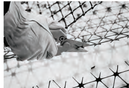
Image 6: Cutting Tensar® TriAx® Geogrid is easily achieved.
