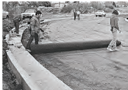
Image 5: Placing Geogrid to accommodate curves.
