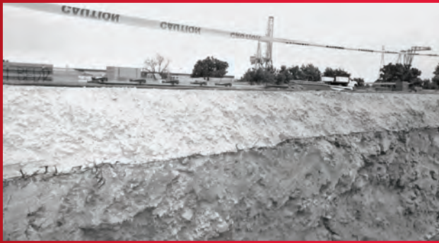
Image 13: A backhoe excavation through Tensar Geogrid.
