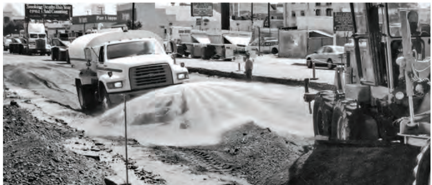
Image 10: Moistening the fill before compaction.
