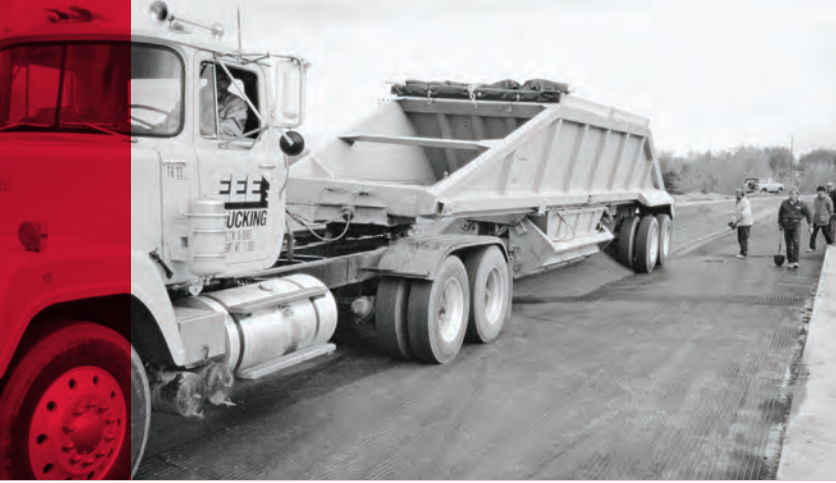
Image 8: Dumping aggregate fill on top of Tensor® Geogrid over competent subgrade.
