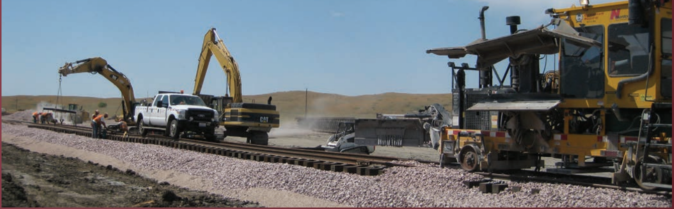
Placing and grading ballast stone on a TriAx Stabilized trackbed
