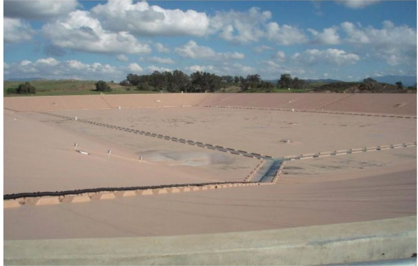
Figure 2. MWDS Skinner Reservoir, CSPE Cover installed 2010
