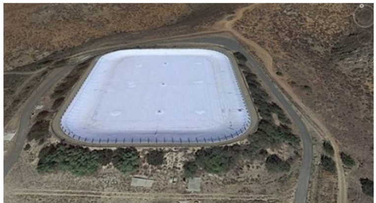
Figure 6. Aerial of Upper Reservoir CSPE Cover
