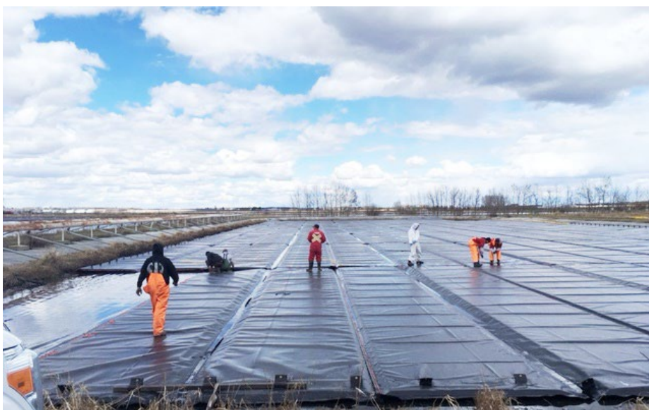
Figure 9. Geosynthetics Technicians walking on the cover during panel deployment
