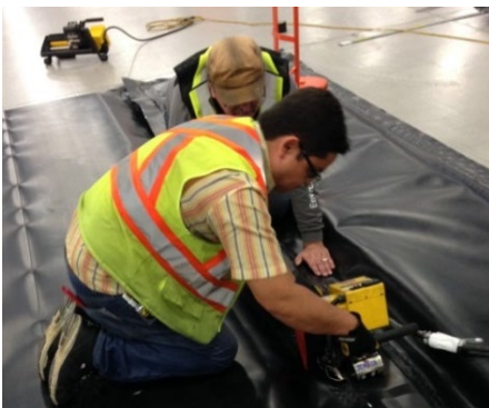
Figure 7. MIC fabrication in the shop
