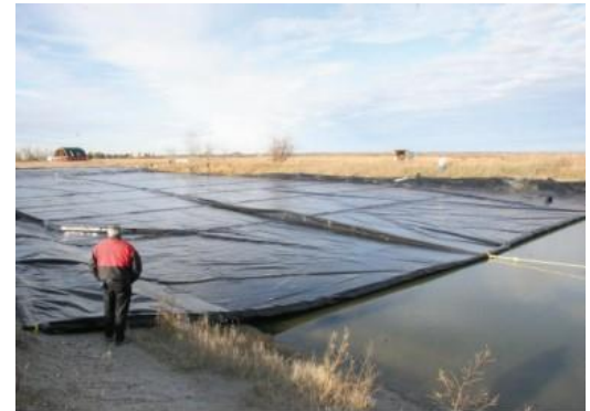
Figure 1. Prototype design lightweight 30 mil (0.75mm) cover system with leading edge
