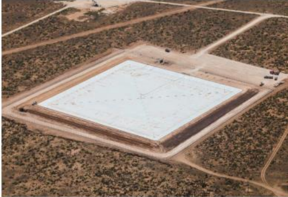
Figure 8. Aerial view of completed 250,000 ft 2 (23,200 m 2 ) Frac water pond evaporation cover in TX.
